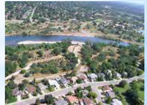
Corps Levee Work
