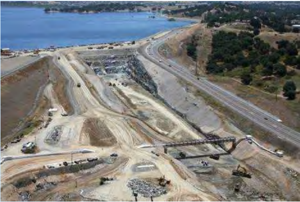
Folsom Dam Project
