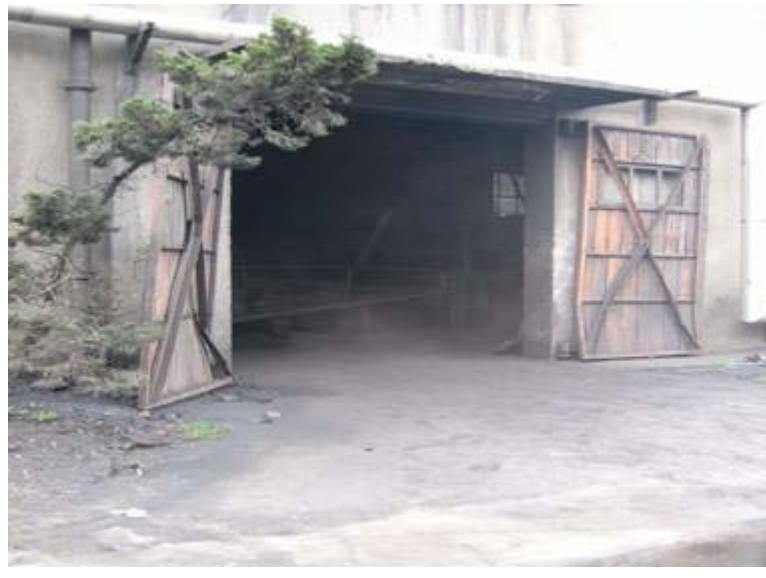
Operation room of the conveyor belt
